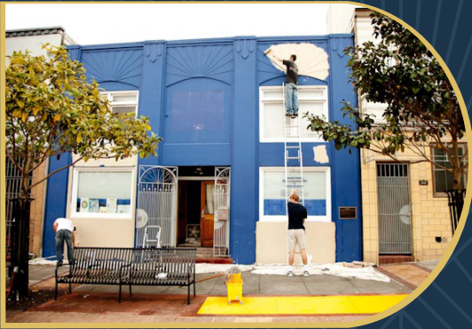
Renovating the restaurant
